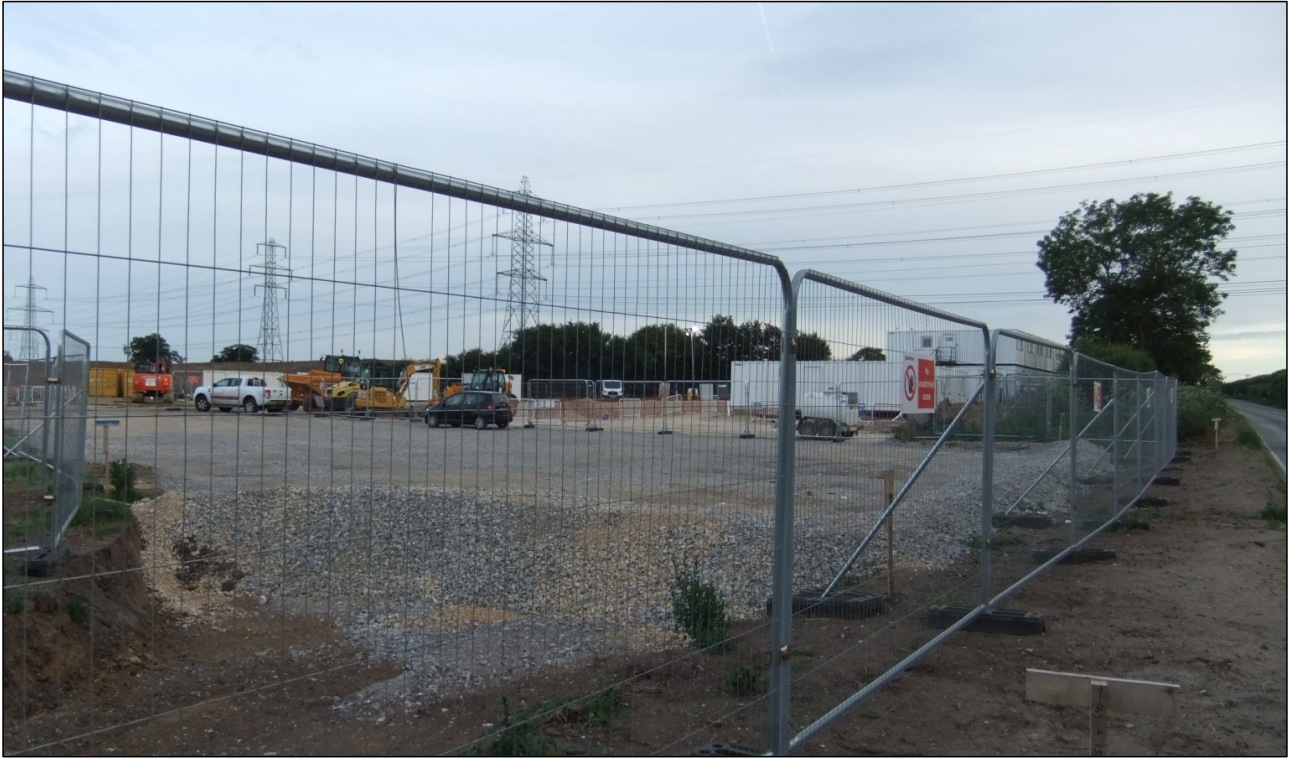
Figure 5: Hornsea Three car park alongside the B1113
