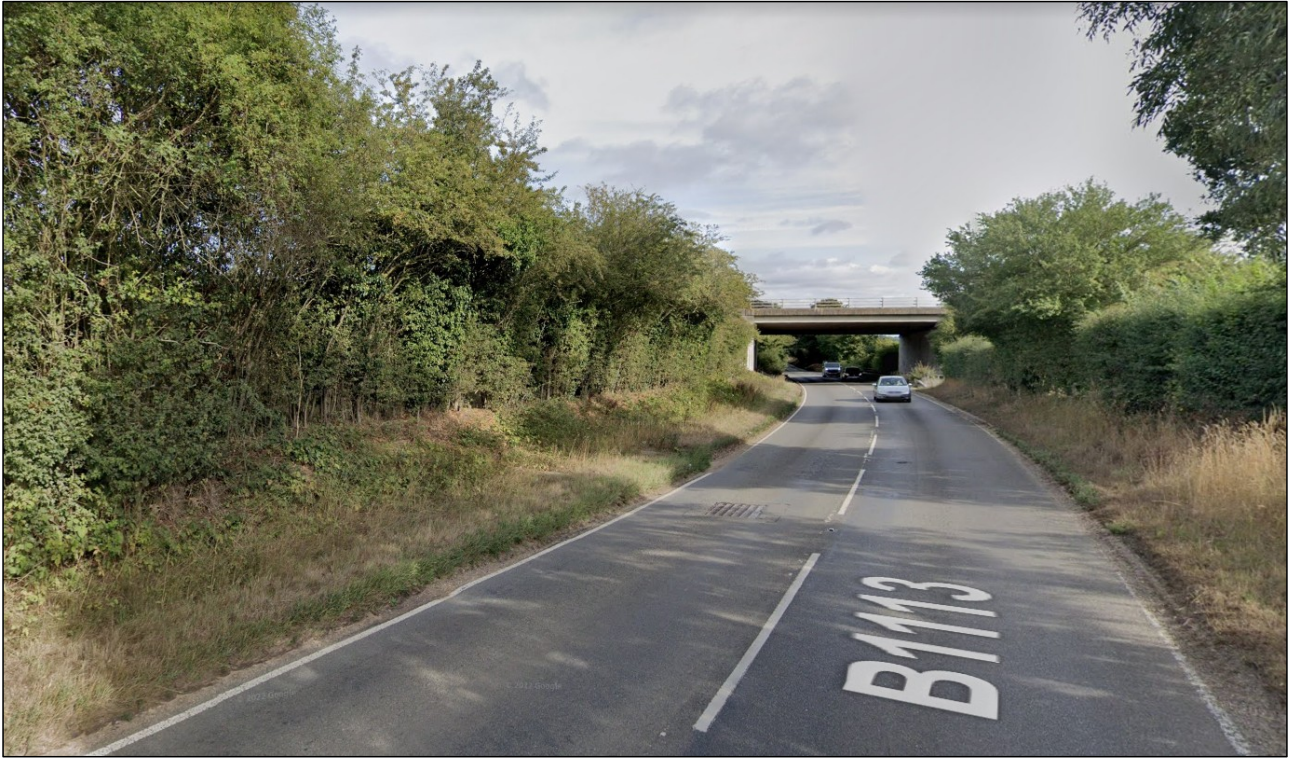
Figure 1: View looking north towards the Southern Bypass
